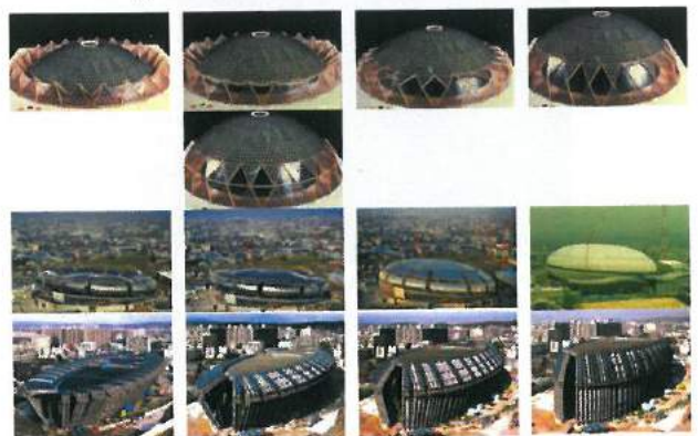
Fig. 14. Idea of Pantadomes. Namihaya Dome & Narahall. From presentation of Mamoru Kawaguchi. LSCE 2005.
