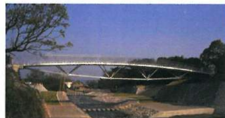
Fig. 8. General View of "Inachus Bridge" with natural stone upper chord. M. Kawaguchi, LSCE 2005.
