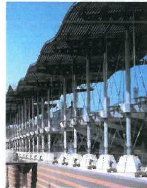
Fig. 7. Prefabricated prestressed concrete piles for compressive members (columns). M.Kawaguch, LSCE 2005.
